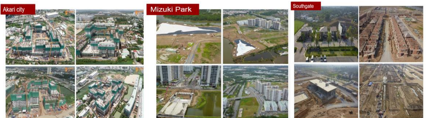
Fig 9: Updated construction progress
